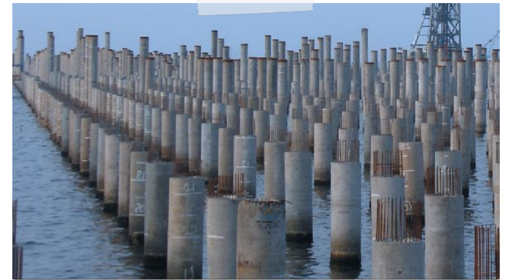
PRE-STRESSED CONCRETE PILES
