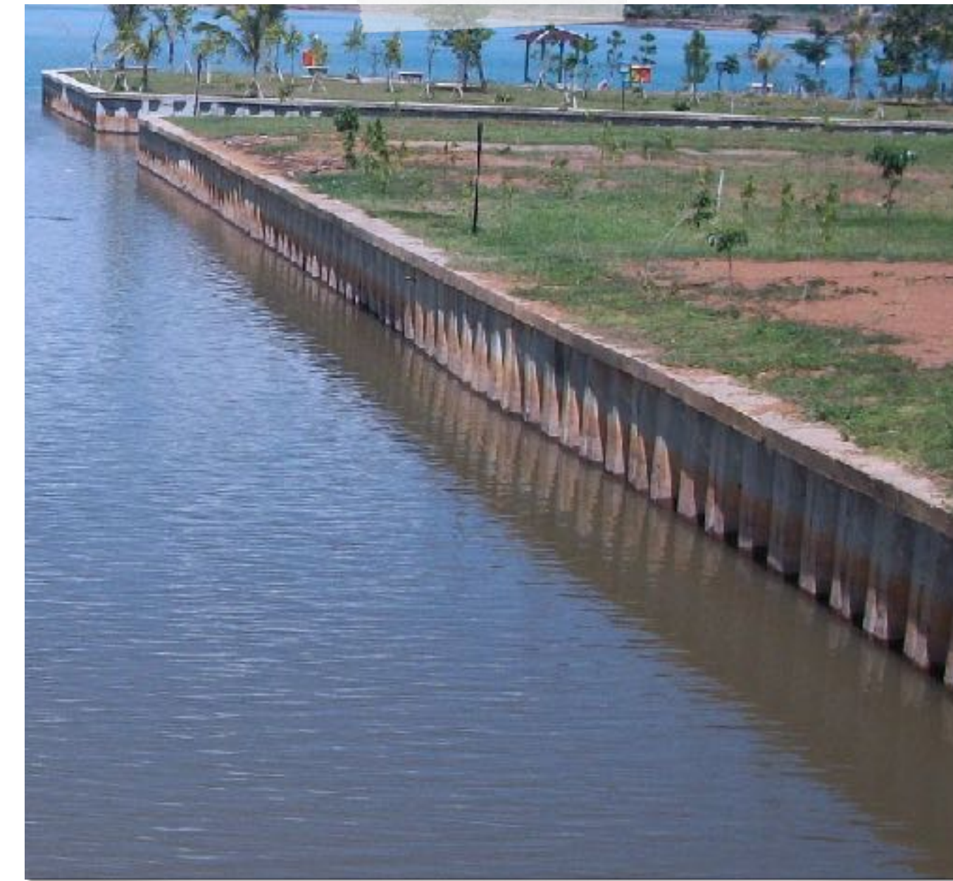
RETAINING WALL CONCRETE
